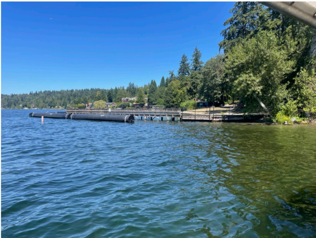
Photo 6 - Shoreline conditions north of the site.
